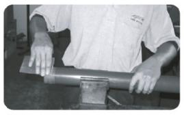
3 Abrade the end of the pipe over the length equal to the socket depth.
