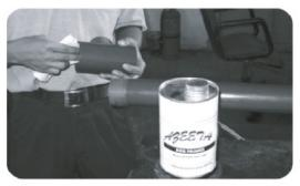
4 Clean the abraded surface with a clean rag moistened with A3EE7A® Primer.
