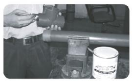
5 Apply A3EE7A® Solvent Cement to the abraded surfaces of the pipe and fitting.
