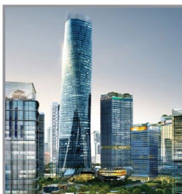
The Exchange 106 (formerly TRX Signature Tower)
